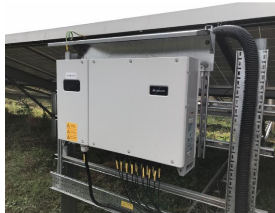
Typical string inverter (image reproduced courtesy of Huawei)
